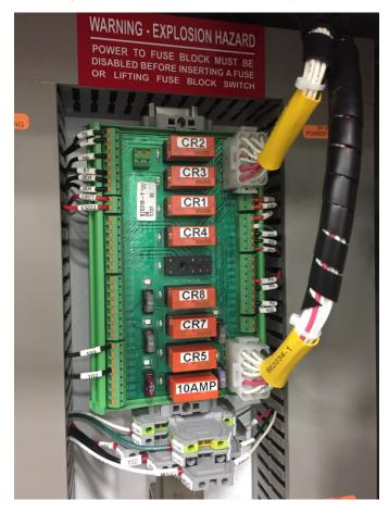
under it to allow the use of a wire tie to hold the relay in place should the unit be installed in a higher than normal vibrating environment.
